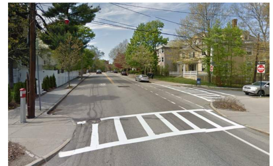
Upper Washington Street – existing condition
